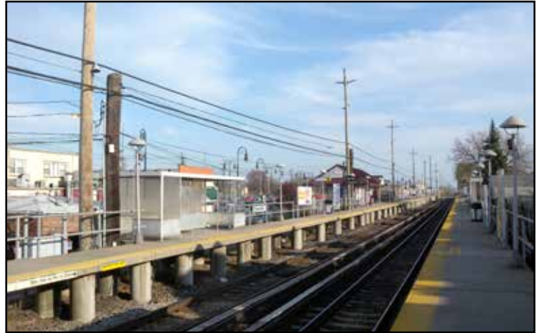
Oceanside Station on the Long Island Railroad, which connects Long Island to New York City. Photo by Jim Henderson.
